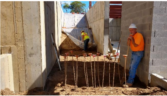
Lower Level Entrance & Stairs Graded
